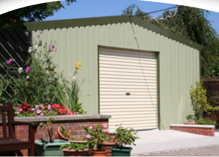
8m x 6m Storage building
