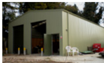
10m x 20m Machinery store
