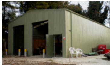
10m x 20m Machinery store
