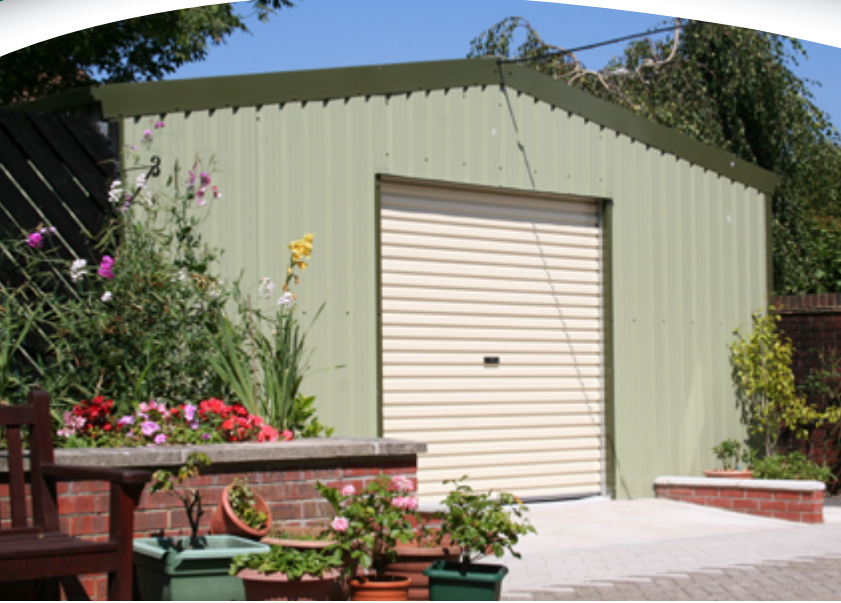
8m x 6m Storage building
