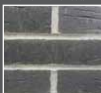
Brick Front Posts
